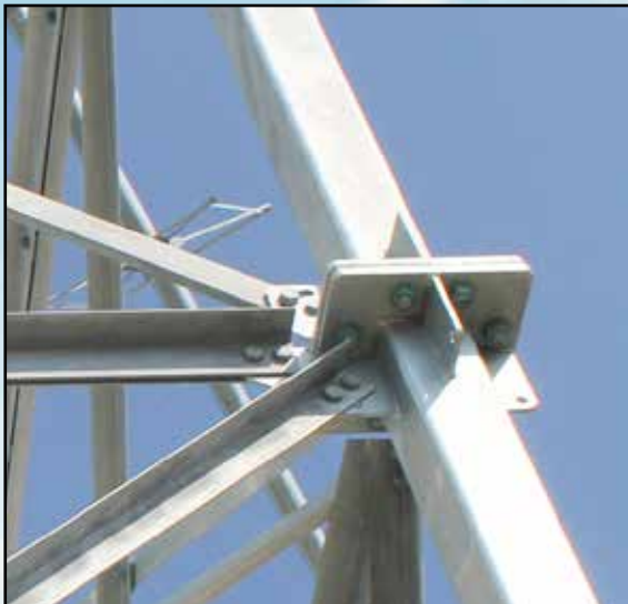
Tower Leg Section Connections
