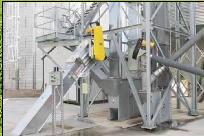
V Bracing for Conveyor Access to Elevator Boot
