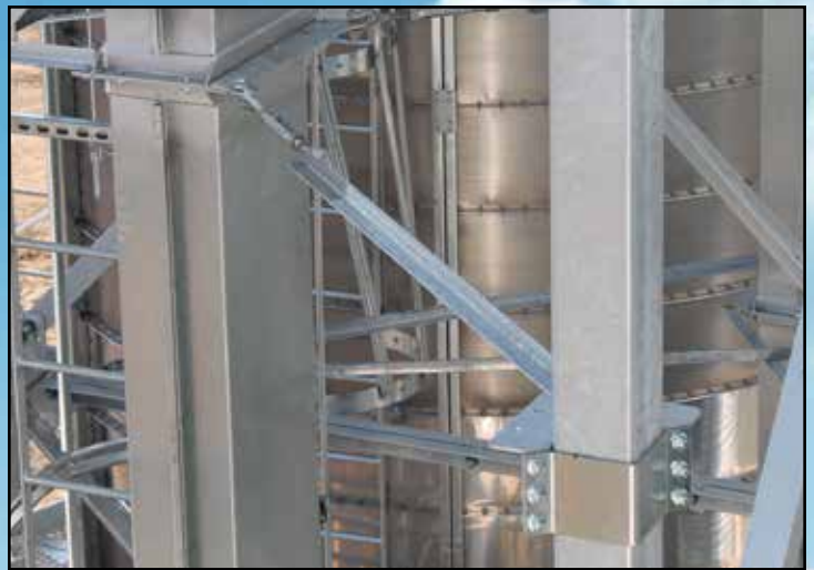
Adjustable Elevator Tie Brackets
