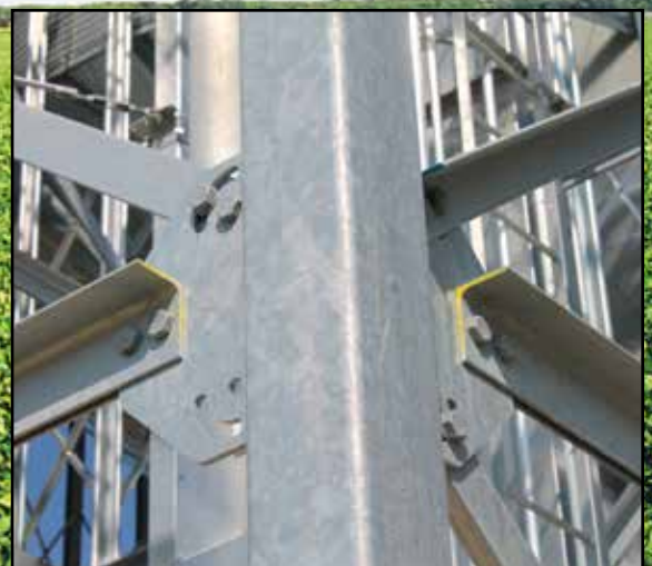
X and V-Bracing Brackets
